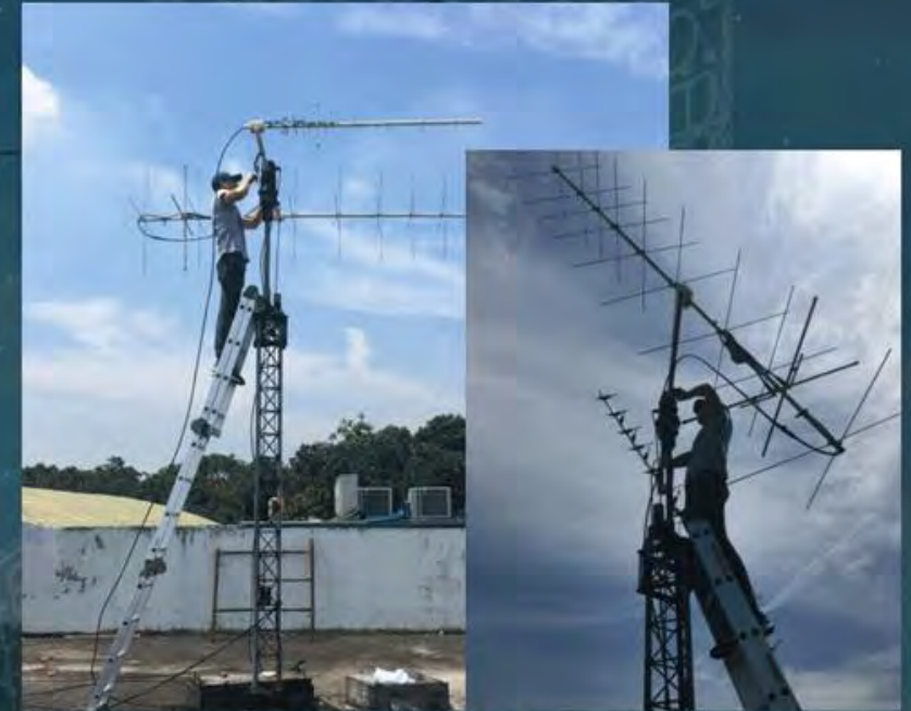
Installing the UHF at the antenna mast
