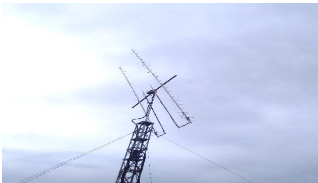
The elevation rotator head seemed to hit the vertical pole
