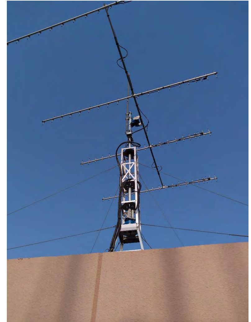
SPATIUM Yagi antenna on rooftop: This is not for the amateur band.
