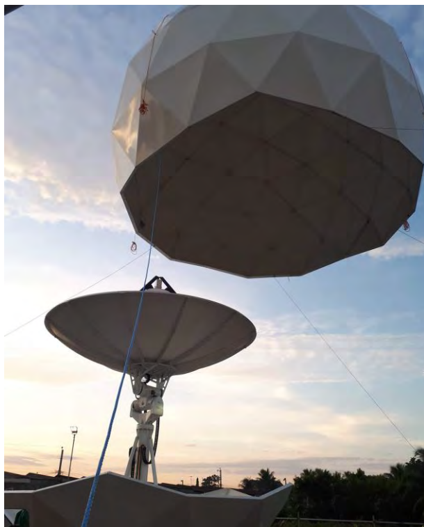
These are photos taken during the construction of the Davao Ground Radio Station in Davao City, Philippines.
