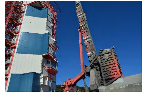
The launch pad after launch
