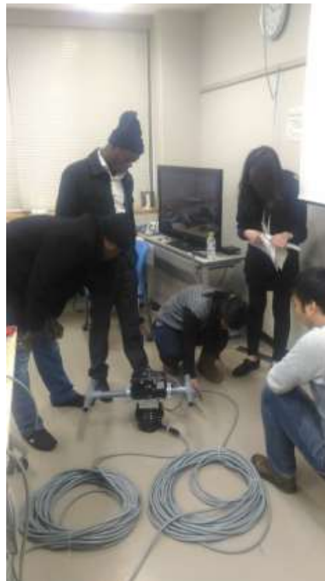
Installing antenna rotator
