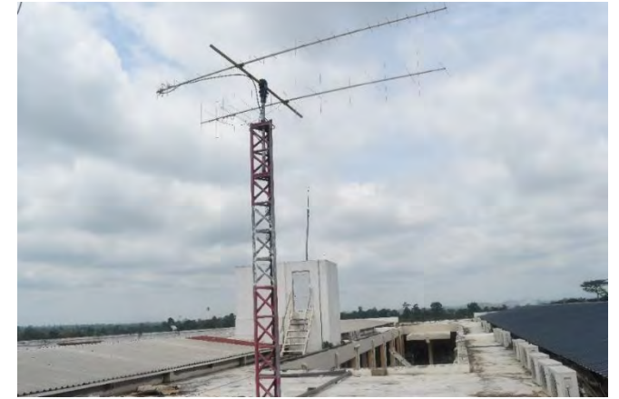
Roof Top UHF/VHF Antenna located at the ANUC Main Campus
