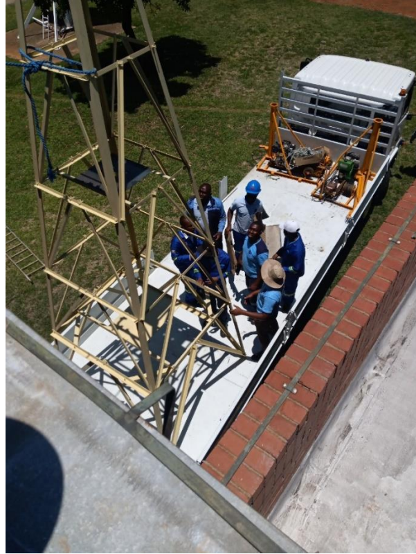
b) Mast being prepared for hoisting
