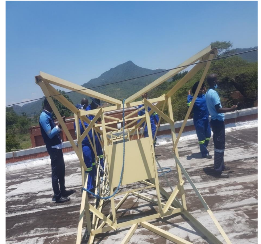
c) Mast hoisted onto the rooftop
