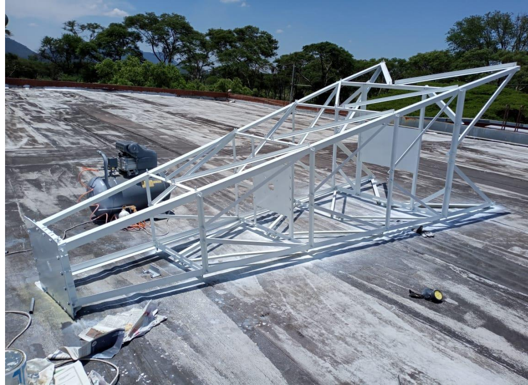
Figure 4) Mast after first white coat was applied
