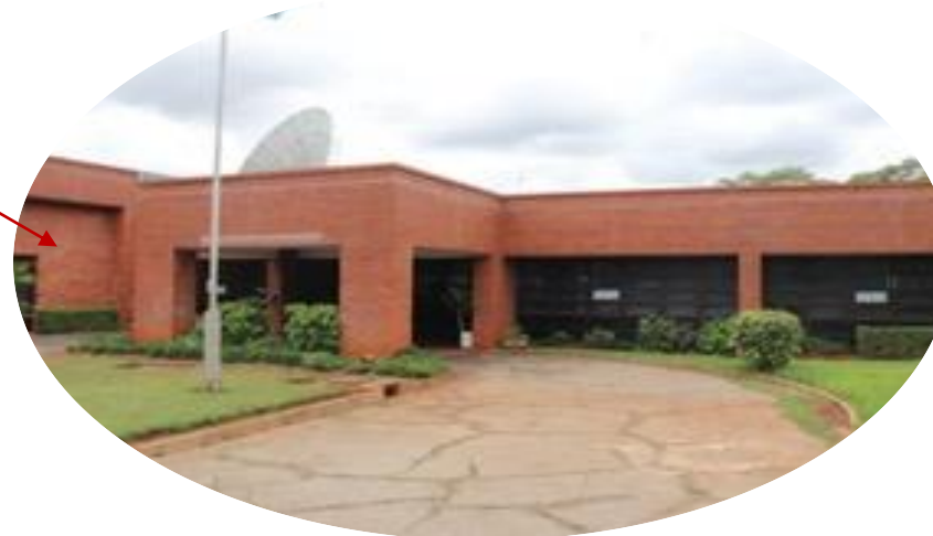
Figure 6b) Outside view of Control room
