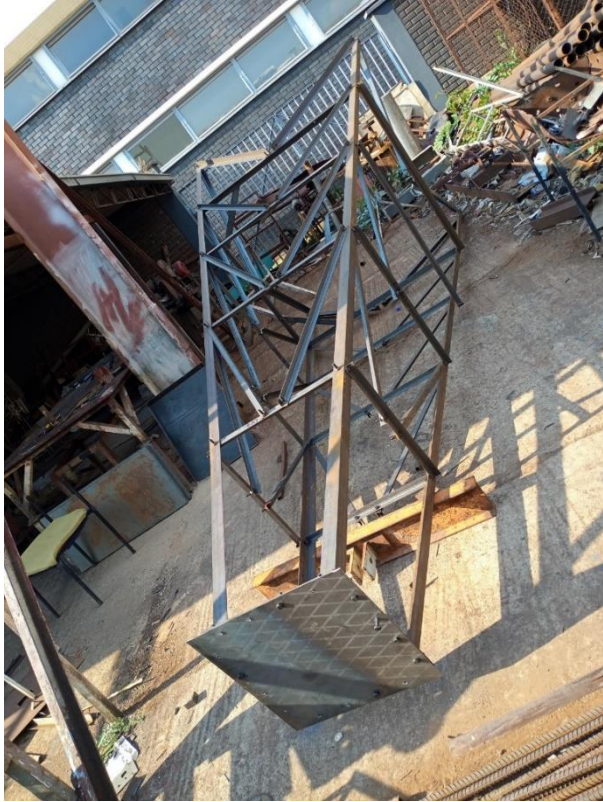
Figure 3 a): Assembling of mast
