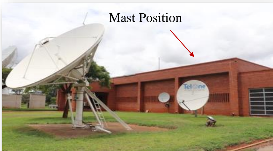
Figure 6a) Mast position on rooftop
