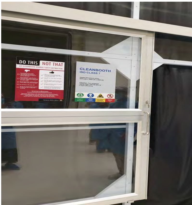
Figures 7: Clean booth inside the AIT facility of MYSA is equipped with blackout static curtain.
