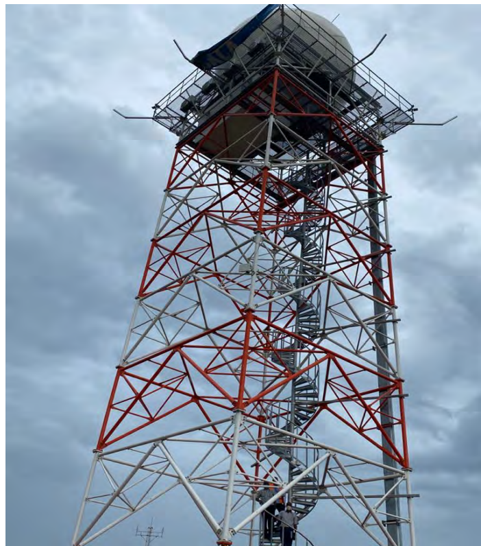
Radar Station – part of the national weather observation infrastructure stock
