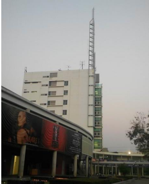
GS antenna is installed at the School of Communication Arts Building.
