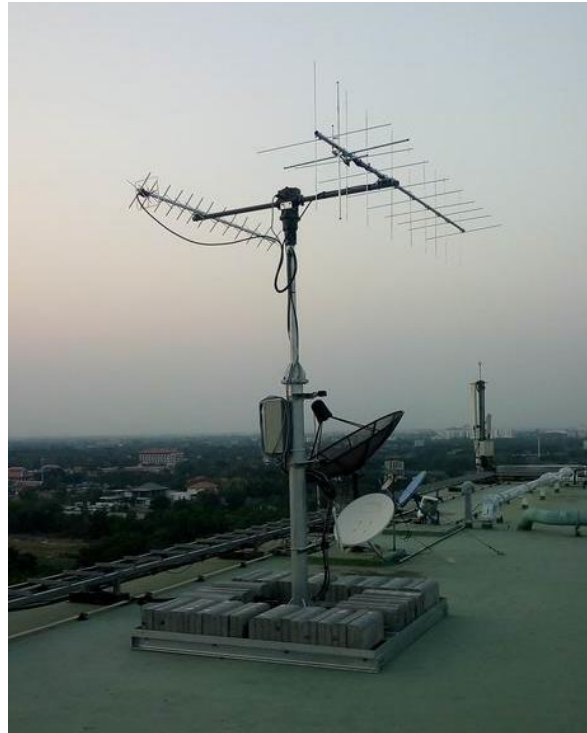
VHF/UHF Cross Yagi-Uda Antenna (on roof of the building).
